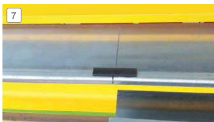
Mounting the joint connector
