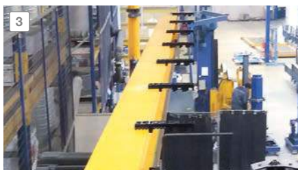
Laying the permanently laid cables
