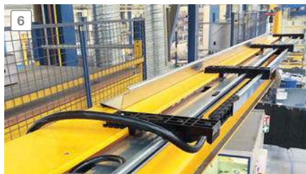
Installation of the cable carrier
