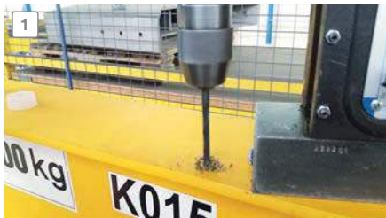
Drilling the mounting holes or mounting the weld-on bolts
